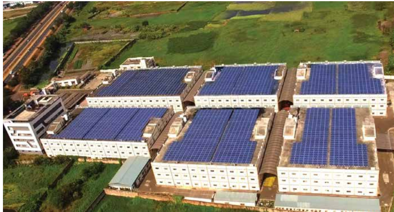
Installed solar panels in the Dankuni factory
