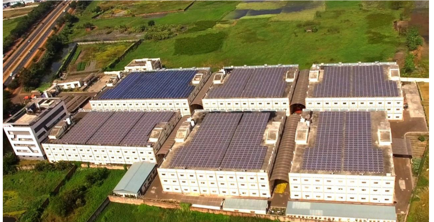
Rooftop solar power plant at Dankuni unit
