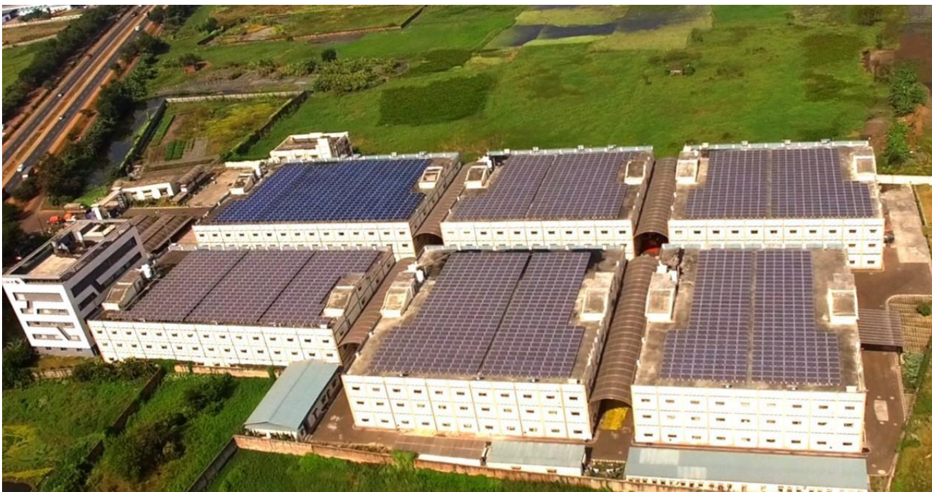
Rooftop solar power plant at Dankuni unit
